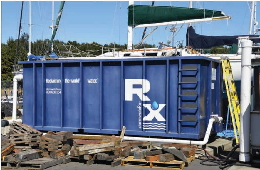
The company invested in a StormwaterRx water-filtration system for the outside yard.
